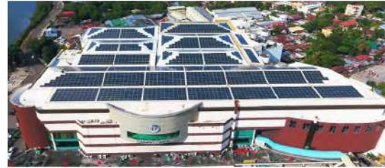
Project Location: Cebu, Philippines Capacity: 2.5MWp Completion Year: 2017 Type: Metal roof Mounted
