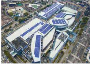
Project Location: Cebu, Philippines Capacity: 2.5MWp Completion Year: 2017 Type: Metal roof Mounted
