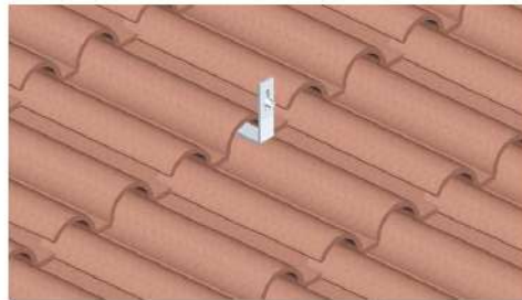
Step 2: Re-instate the Tiles
