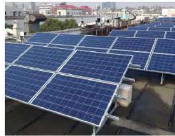
Project Location: Shanghai, China Capacity: 4.3MWp Completion Year: 2016 Type: Concrete Roof Mounted
